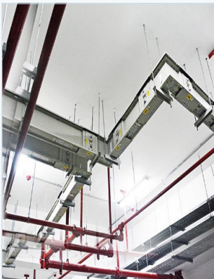
Example of a horizontal busway installation along the ceiling 9
